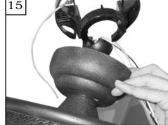
Raise fan with downrod assembled to the ceiling bracket and hang fan assembly. Be sure to rotate the downrod ball so that the notch in the bracket engages the slot in the ball.
